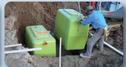
Installazione impianto Depurfamily® Installation of Depurfamily® plant
